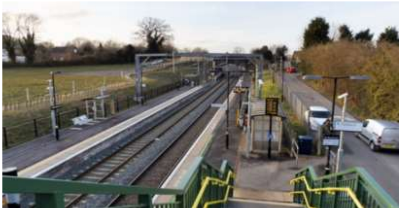
Fig 57. Alvechurch new rail station completed 2015
